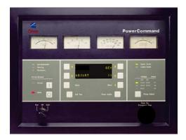
The PCS is a microprocessor based genset monitoring, metering and control system. It is integrated into the GCP2 and incorporates the following key features;
